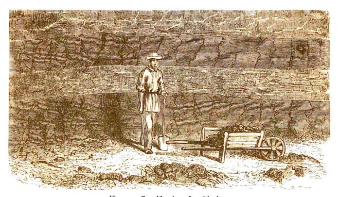
Fig. 70.—Stratification of coal-beds.
